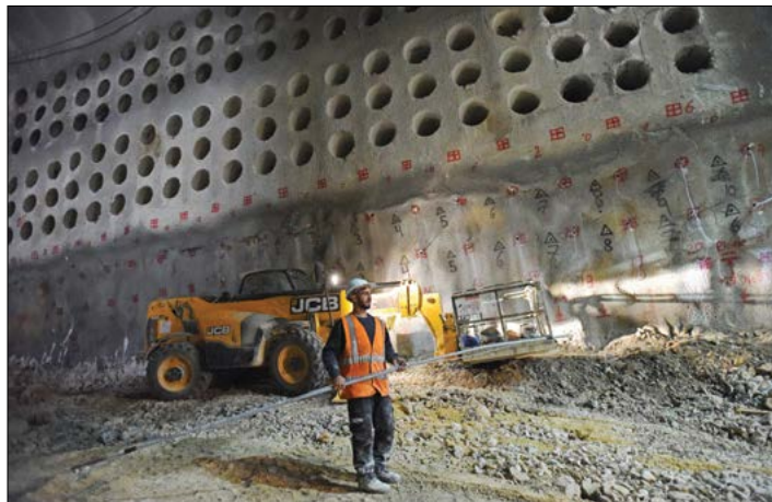
A worker carries material under burial niches in the wall, where bodies will be buried, in the underground cemetery project under construction.
