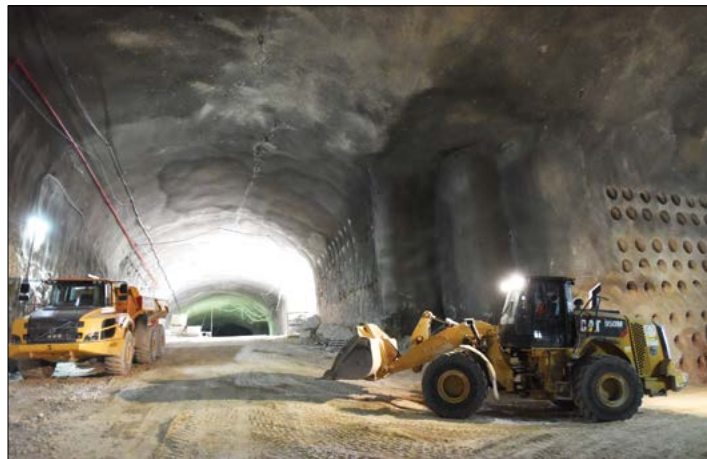
Construction is in progress to build the underground addition to Har Hamenuchot Cemetery, which is a half-mile long and 164 feet deep, the height of a 15-story building.
