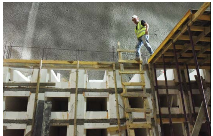
A worker walks on top of precast graves under construction in the cemetery project.
