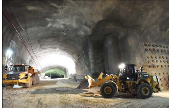
Construction is in progress to build the underground addition to Har Hamenuhot Cemetery, which is a half-mile long and 164 feet deep, the height of a 15-story building.
