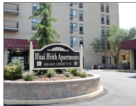
B'nai B'rith Apartments in Allentown, Pa. (one of the first 202 buildings sponsored by B'nai B'rith). First established April 1979, 151 apartments funded under Section 202, 120 apartments added: established January 1983.
